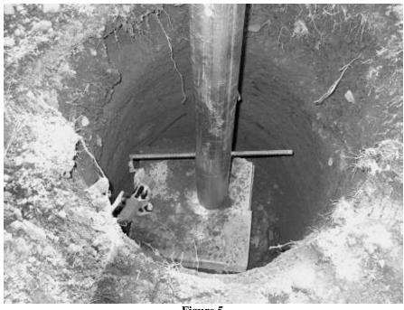
Figure 5 Mast are set on concrete blocks in each hole, with reinforcing bar to prevent twisting (see text).
