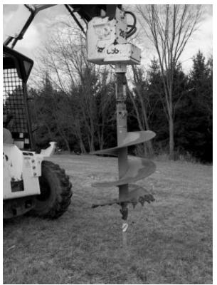
Figure 4 Auger being aligned on first antenna location stake.
