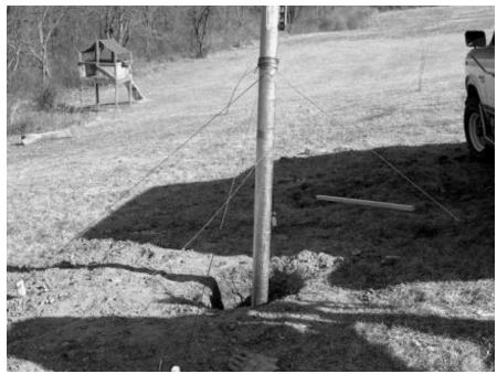
Figure 8 Temporary guys hold the masts in position during the pouring and setting of the concrete.
