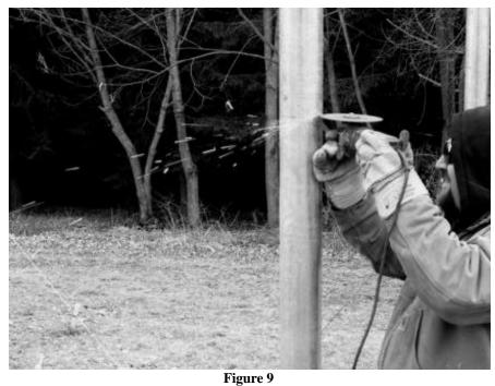
After measuring with a string level, all eight masts are cut off to the same absolute altitude.
